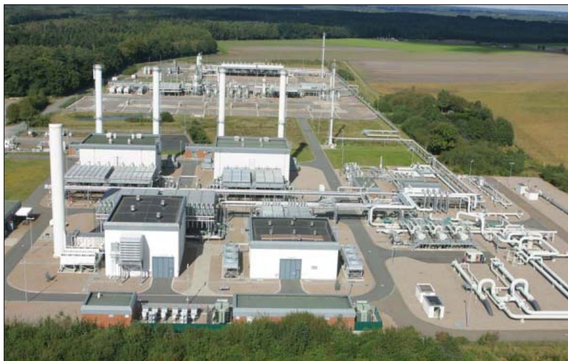
With only 16 wells for its 7 billion cu m capacity, Rehden uses horizontally drilled wells tied back to this central location for injection and offtake (Fig. 1).
